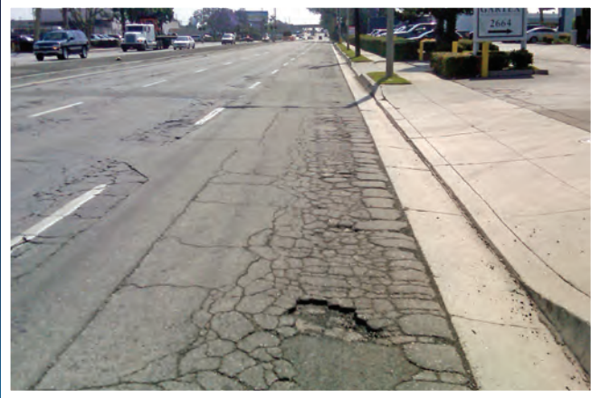
(Above) Pre-Condition - Close-up – Severe alligator cracking along existing edge of gutter (pop-outs).
