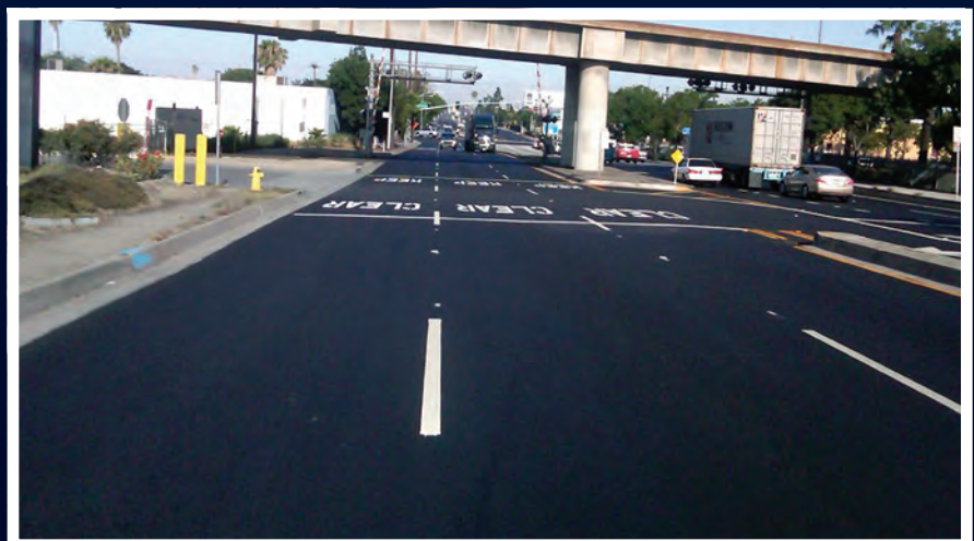
(Below) Post-Condition – Final rubberized asphalt paved roadway.
