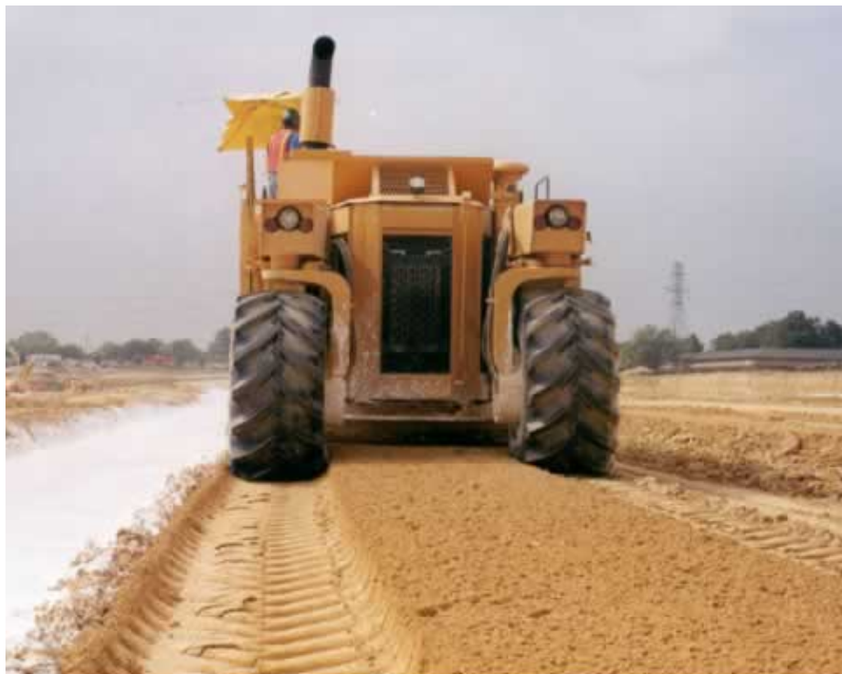
Figure 14: Rotary mixer used for initial mixing
