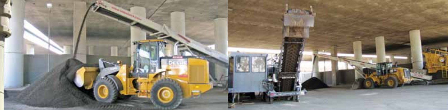
Above: Stockpiled RAP being processed as CCPR at the recycling site provided by the City of Glendale. After recycling with the engineered emulsion, the asphalt is loaded into trucks for subsequent delivery to the paving operation.
