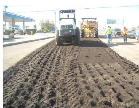
FORTRESS APPLICATION AND COMPACTION
