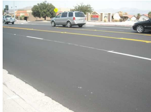
FINISHED PRODUCT WITH 1.5" HMA OVERLAY
