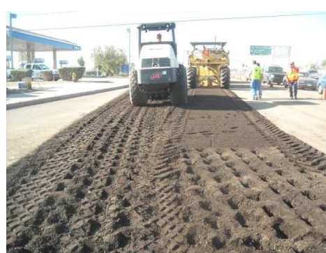
FORTRESS APPLICATION AND COMPACTION
