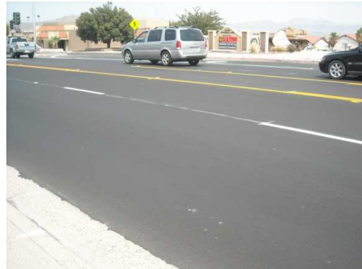
FINISHED PRODUCT WITH 1.5" HMA OVERLAY
