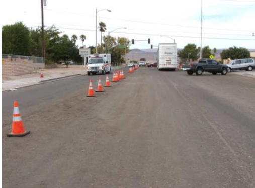
AFTER COMPACTION AND TRAFFIC RELEASE
